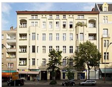
Apartment building at Hauptstraße 155, Schöneberg , Berlin, where Bowie lived from 1976 to 1978
