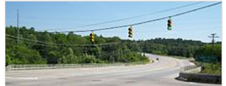
James Taylor Bridge, Chapel Hill, North Carolina
