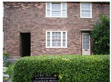
The home at 20 Forthlin Road in Allerton , into which the McCartney family moved in 1955
